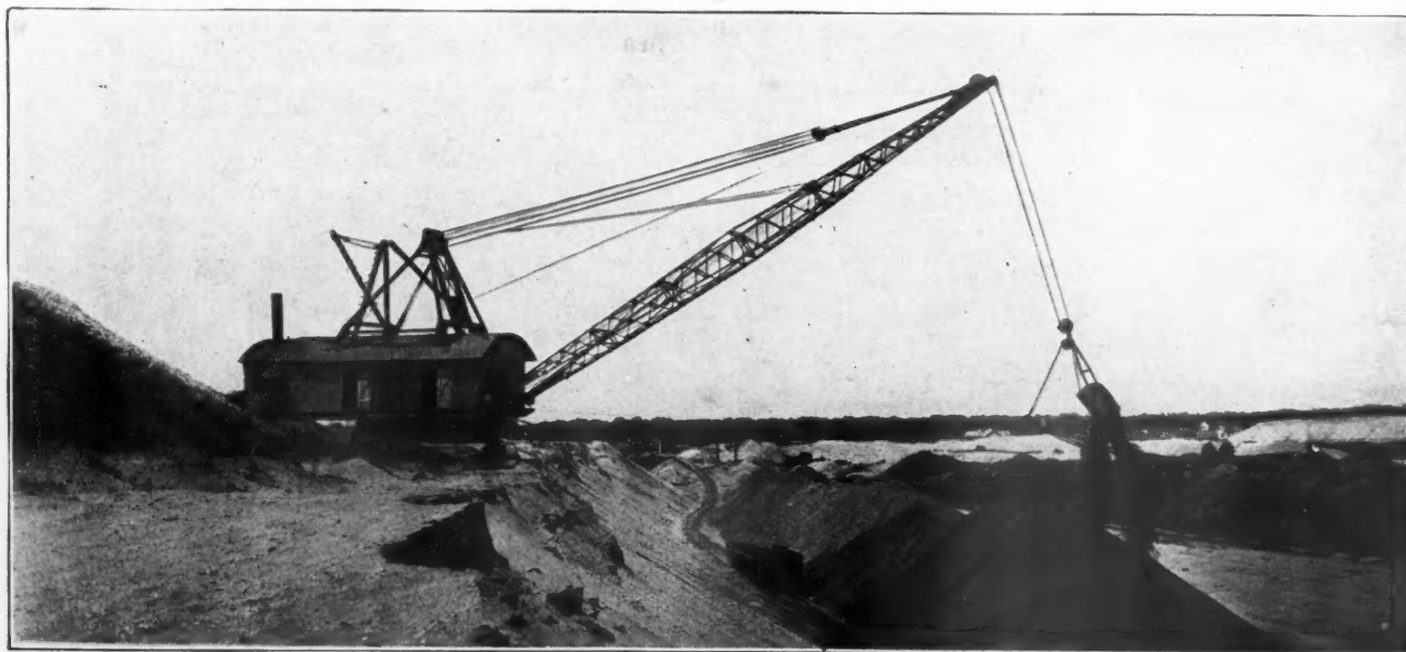
View of Stripping Operation
